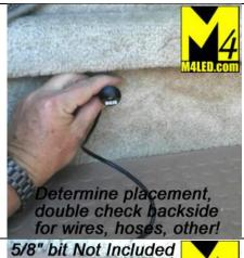
Every Installation is Different. The following are general guidelines for installation, not specific details. Basic 12 Volt DC wiring is required.
