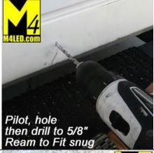
• Drill a pilot hole. Check again behind the hole that there are no obstructions, the exit point will be easier to see.
