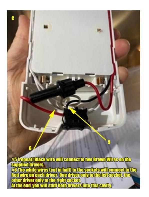
The Black Wires from the drivers need to go to the sockets at the other end of the fixture.
